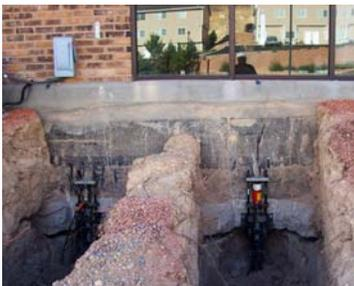
There was minimal disturbance to the building's occupants during the restoration process. Because ECP Steel Piers™ were installed using quiet, vibration free hydraulics, it was "business as usual" in the office during the underpinning installation.
